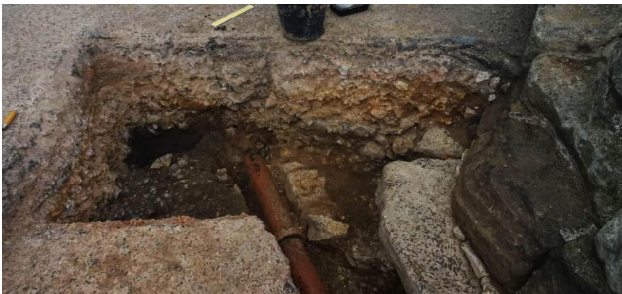
Photograph 6 (08 August 2016). View of Section 3, with evidence for cut 2 (F3) destruction: note the dark clayey [28]/[29] on left has no equivalent on right. The upward curve of [25] at the cross end of the section is clear. F1 (right of pipe) clearly had no more courses.
