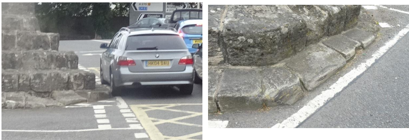
Fig 2: Left: BMW hits Congresbury cross, July 2016 Right: Scuff mark from above (among earlier collision marks). Note the damaged nature of the edge of all the roadside stones (not seen on other sides of the cross)
