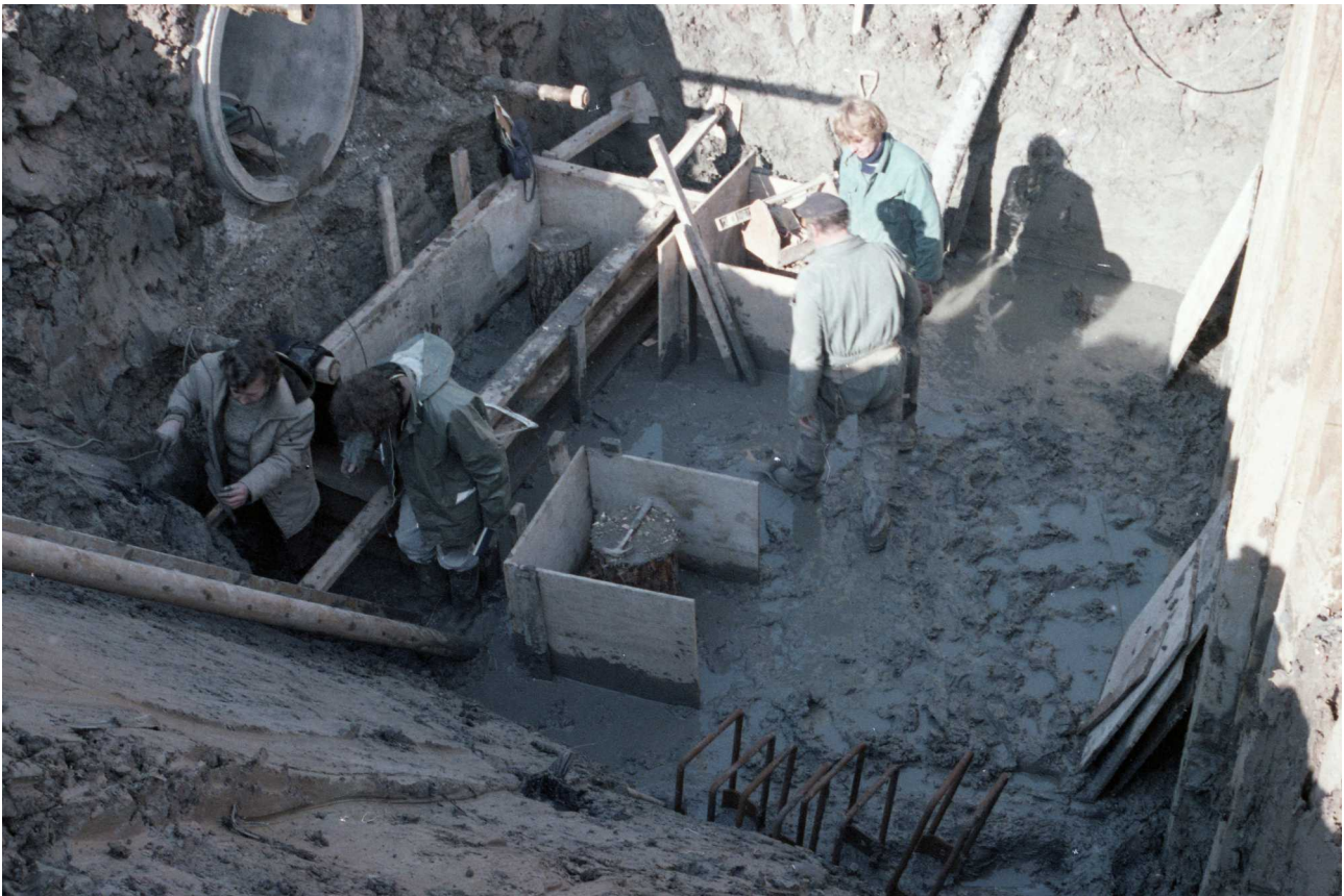
Salvage recording on site amid preparations for concrete pouring, 1982
