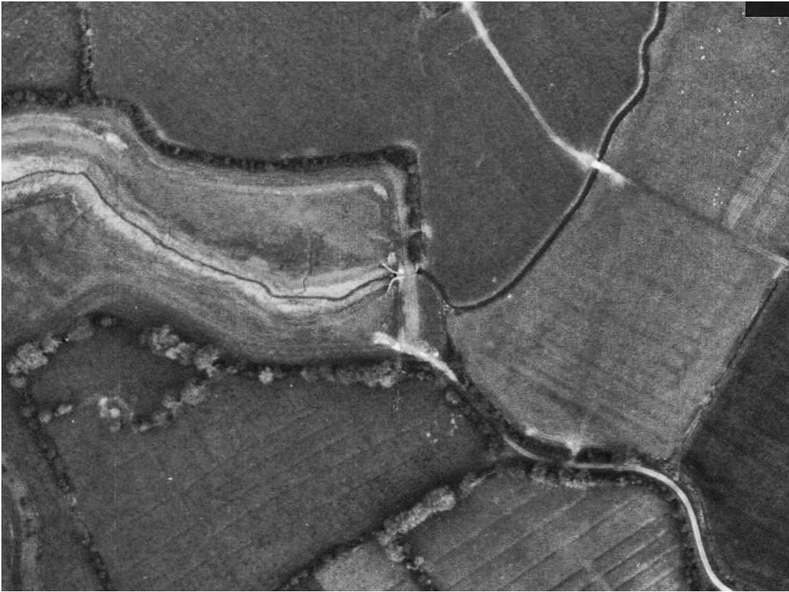
Fig 7: Sluce before 1982 works (North Somerset 1975_9008)
