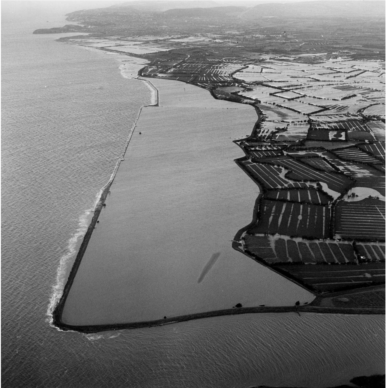
Fig 7: Hurdiches and surroundings flooded in December 1981 (Photographs courtesy of David Crossman).
