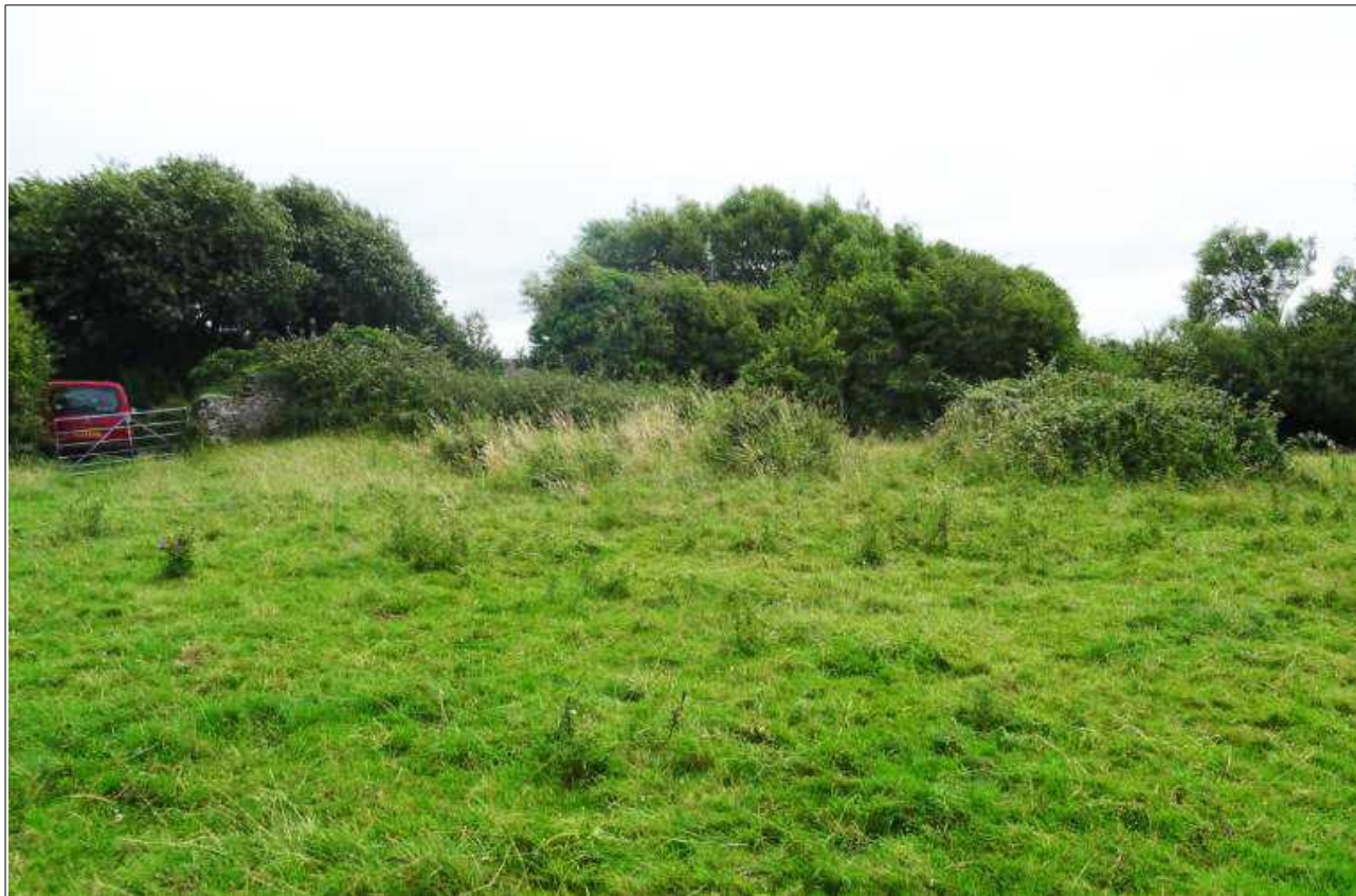
Fig 10: Site before bramble clearance, from west: the brambles are mainly growing on rubble piles from building collapse / demolition
