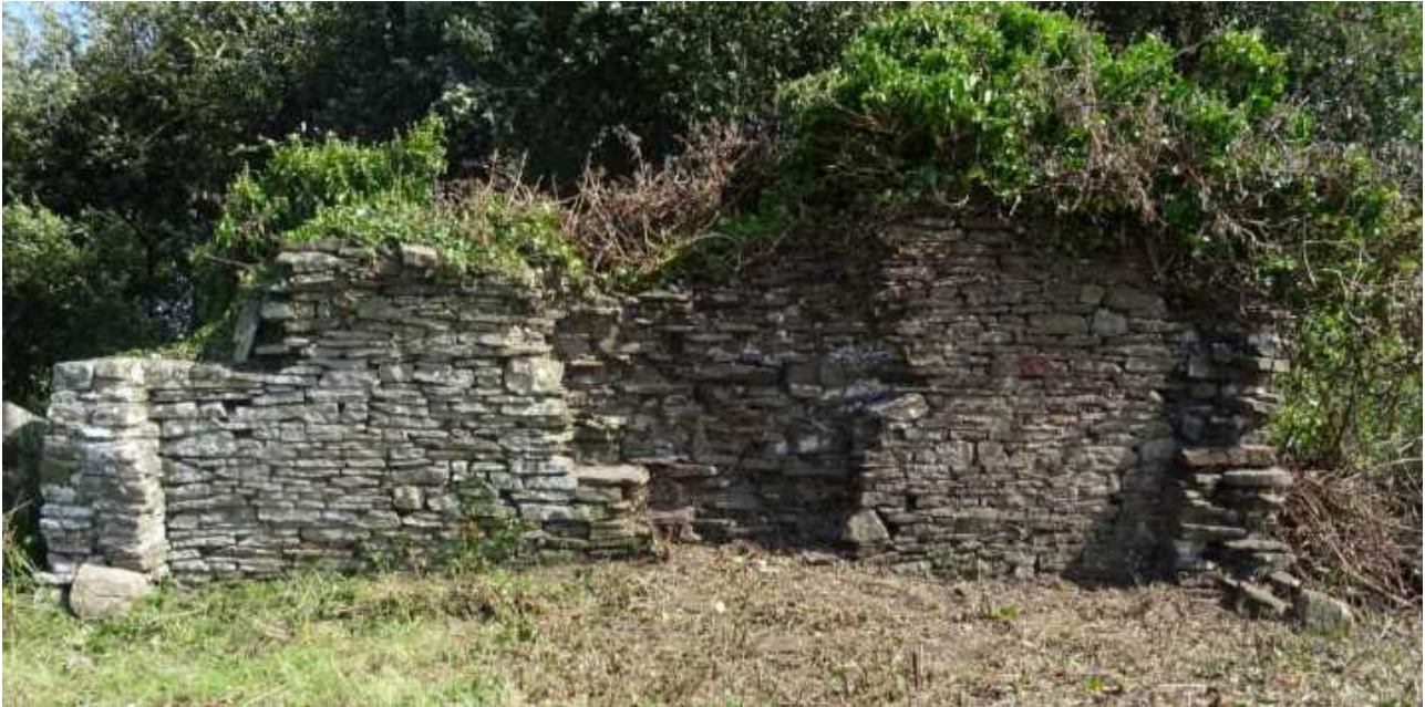
Fig 13: The trackside wall (west elevation)
