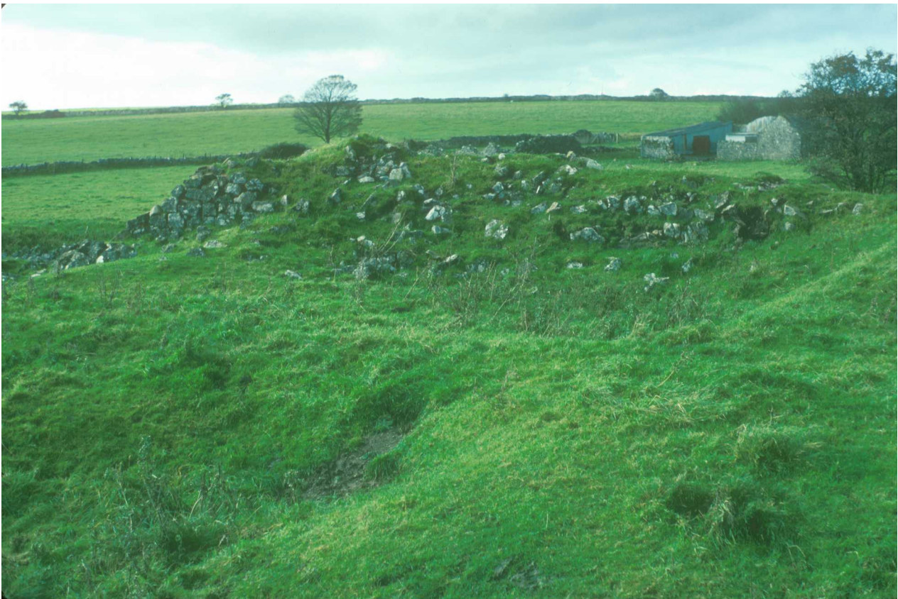
Fig 3: Limekiln (see above) at Milkway: Milkway Barn in background (1988)
