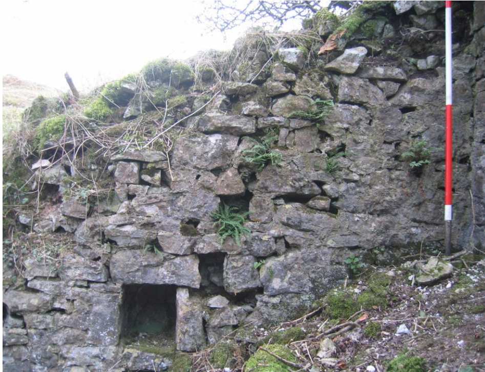
Fig 6: Junction of west cheek wall with kiln face, from E
