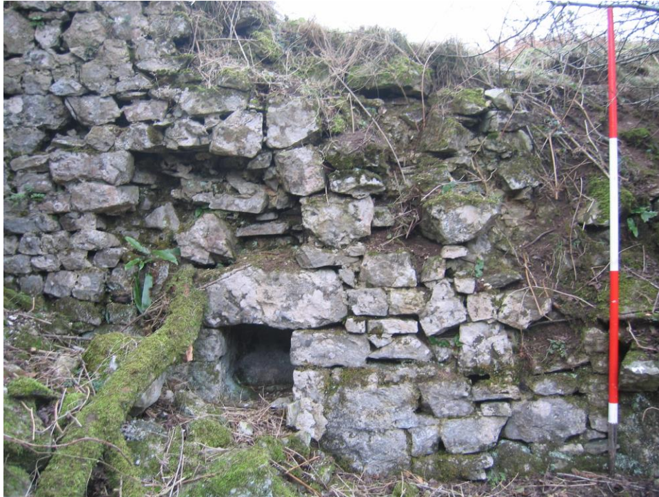
Fig 4: East cheek wall with large recess, from W
