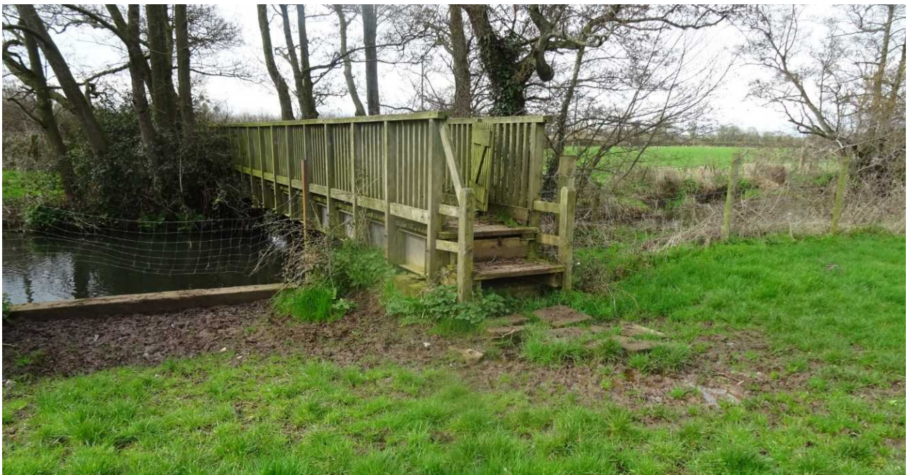
Fig 5: Iwood footpath bridge, 2018
