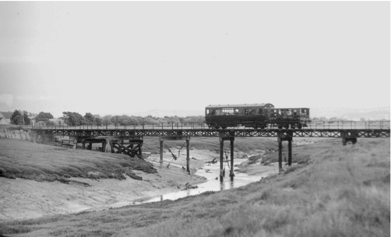
Fig 41: Weston, Clevedon and Portishead bridge in use c1930 (Mitchell & Smith 2003)
