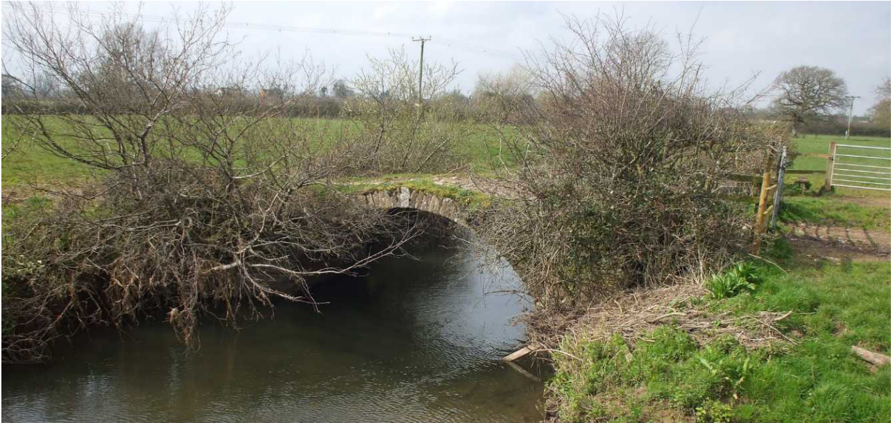
Fig 10: Iwood bow bridge, east elevation 2014
