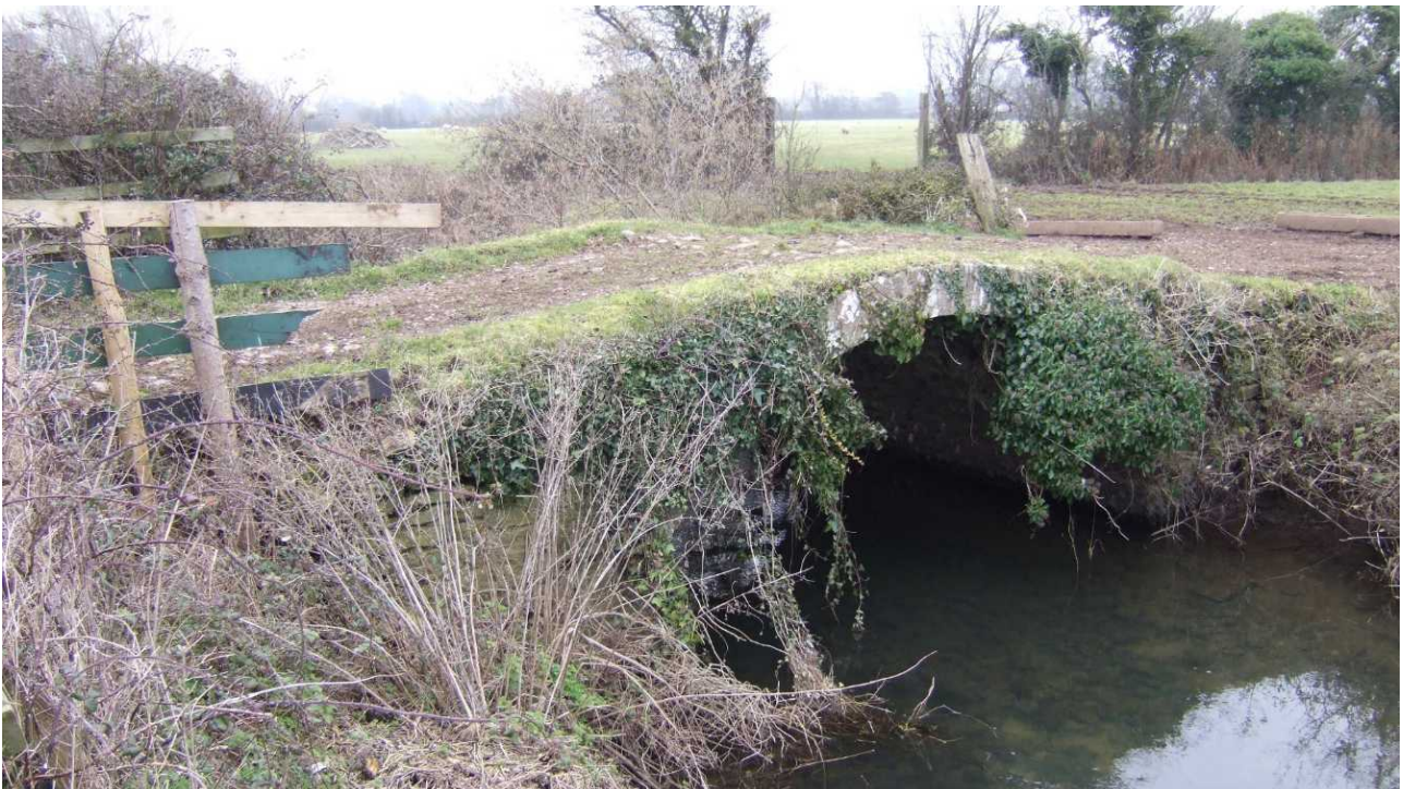
Fig 11: Iwood bow bridge, west elevation 2006
