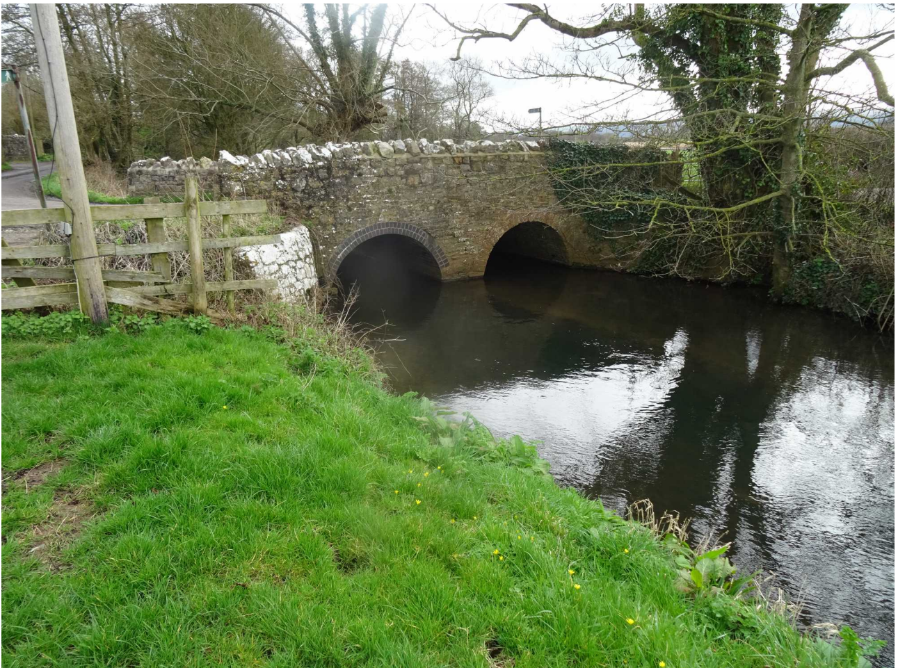
Fig 6: Iwood road bridge from the west, 2016
