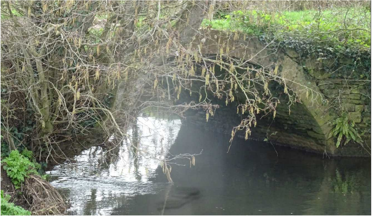
Fig 14: Somerset Lane bridge, west elevation 2014
