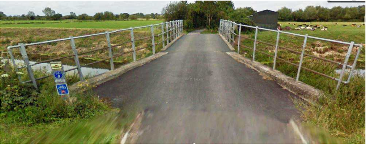
Fig 27: Moor Lane bridge 2022 (Google Earth Street View)
