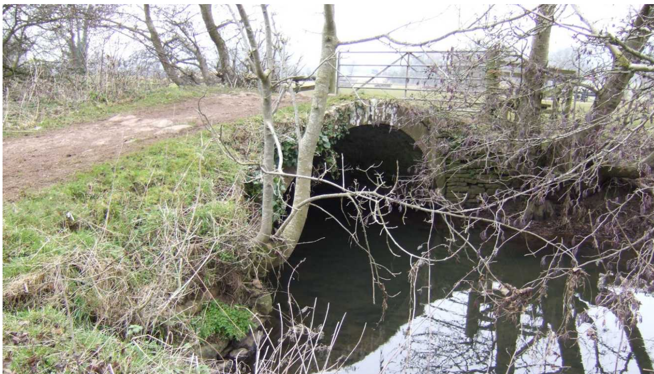
Fig 13: Somerset Lane bridge, east elevation 2006
