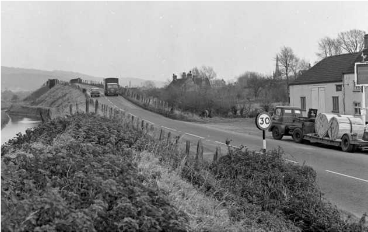
Fig 25: Mid-1960s photograph showing the river crossing already removed, while the road bridge awaits removal.
